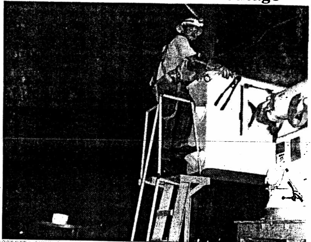
A Guam Power Authority crew fixes a power pole at A. Sanchez in Harmon after a truck accident causing power outage for about four hours in the area.
